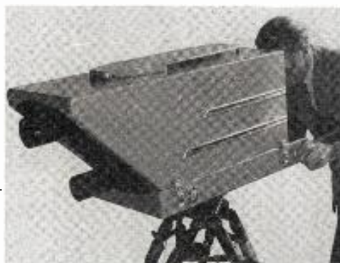
BRITISH-BUILT camera used in live and film High-Definition production and recording, presently utilized by BBC.
